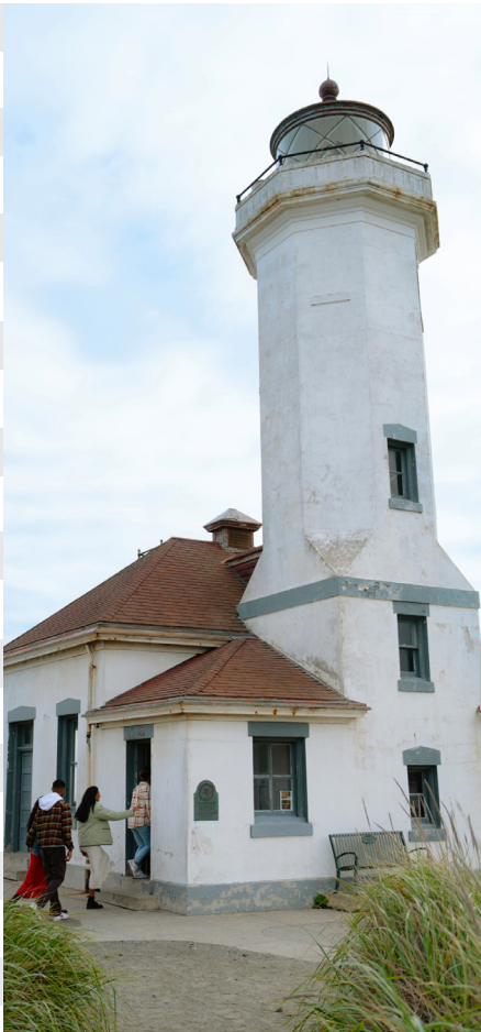
Point Wilson Lighthouse
